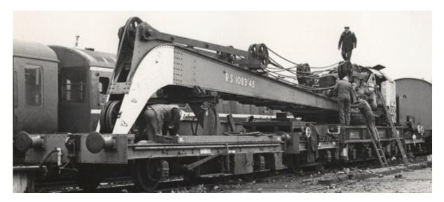
Hoist rope and jib ropes are removed from the jib, which will be craned off for separate movement, the jib runner and the jib travelled to Sussex in that order using the same flatbed lorry over 2 round trips.
