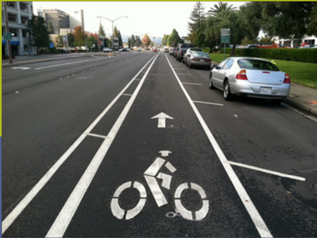
Figure 3-6. Buffered bike lane in Redwood City, Calif. (Image: Silicon Valley Bike Coalition)
