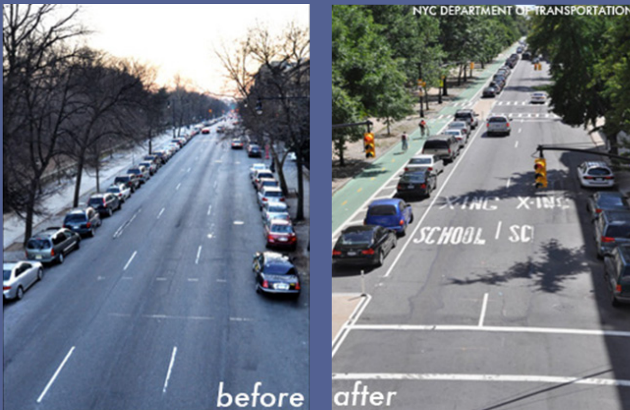
Fig. 3-1. A complete streets redesign of Prospect Park West in Brooklyn, NY added a protected bike lane and pedestrian islands and removed one automobile lane. Before the redesign, 74% of cars were speeding and 46% of cyclists were riding on the sidewalk. After the redesign, only 20% of cars were speeding and only 3% of cyclists rode on the sidewalk. Injury crashes declined by 63% after the redesign and travel time for drivers was not affected. (Images and stats: NYC Dept. of Transportation)
