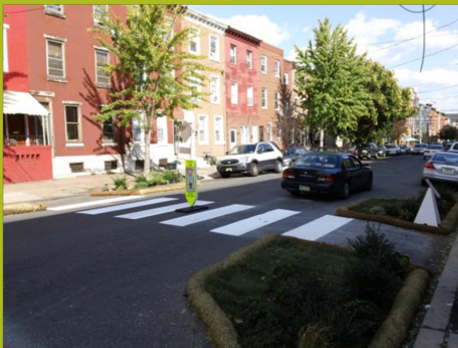
Fig. 3-2. A pedestrian bump-out in Philadelphia using inexpensive materials. (Image: BetterBlock.org)
