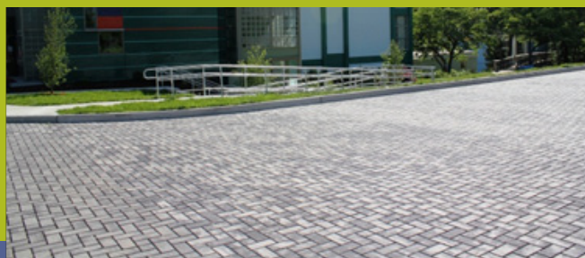
Fig. 5-11. Permeable pavers at the Discovery Museum and Planetarium in Bridgeport, CT. (Image: Save the Sound)
