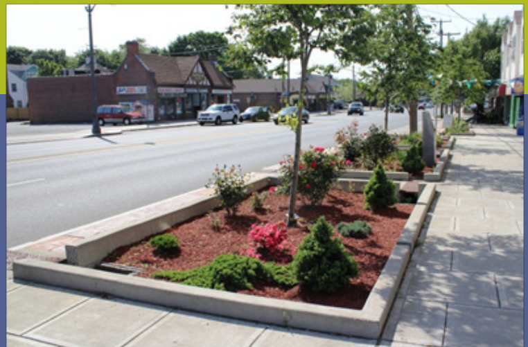
Fig. 5-2. Bioretention bump-out on N. Main Street, Bridgeport, CT (Image: Save the Sound)
