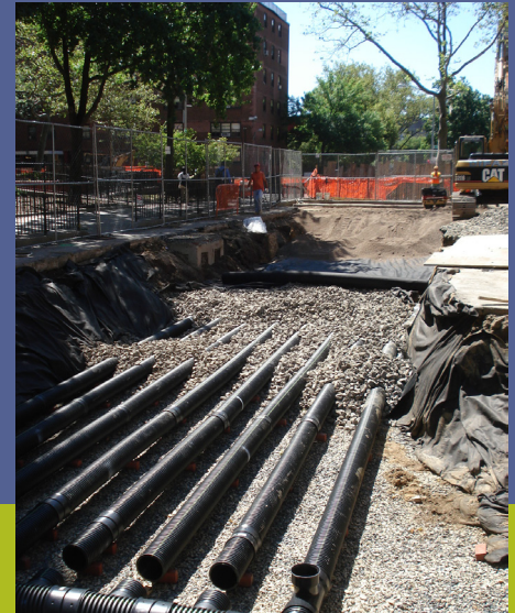
Fig. 5-7. Subsurface perforated pipe infiltration system in New York City. (Image: Hazen & Sawyer)
