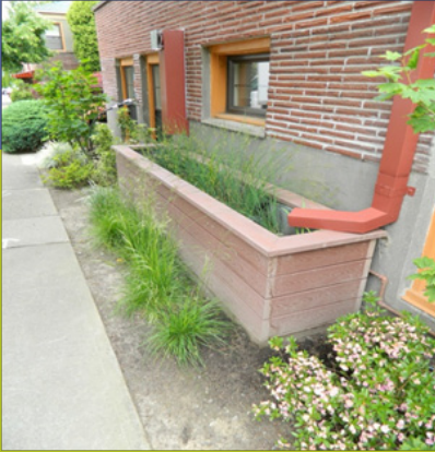
Fig. 5-6. Downspout disconnect into a stormwater planter box (Image: EPA)
