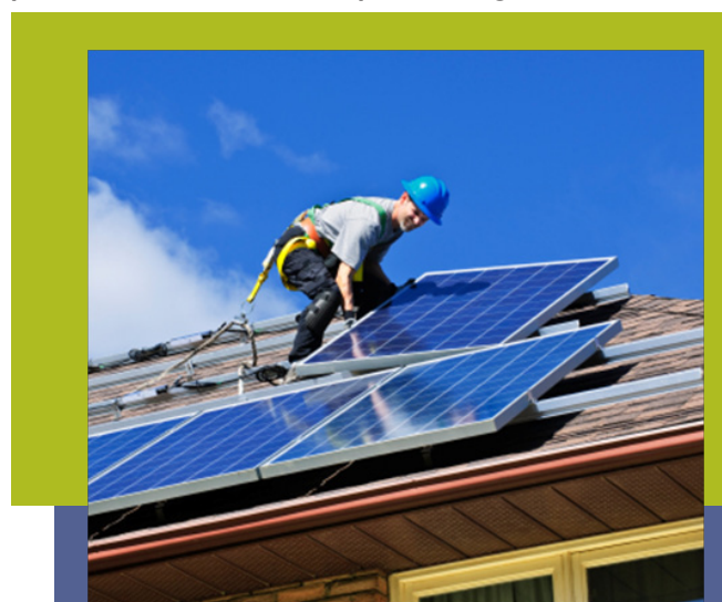
Figure 6-4. Installation of solar panels. (Image: ecooutfitters.net )
