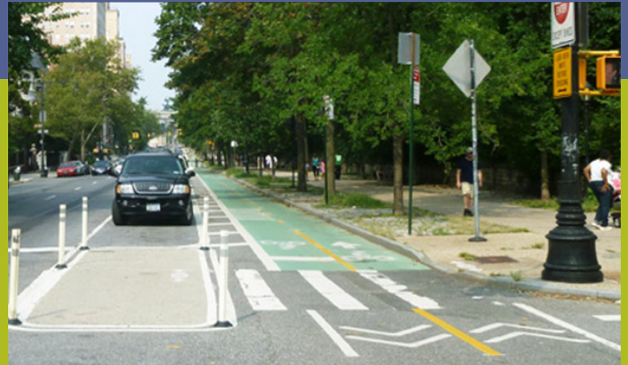
Figure 3-7. Protected two-way bike lane in Brooklyn, NY. Parked cars separate the bike lane from the rest of the street, creating a protected space for cyclists. Bollards or concrete can also be used to physically separate a bike lane. Note pedestrian island at left. (Image: L Magazine)
