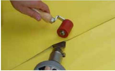
Heat welded CoreFlex seam
