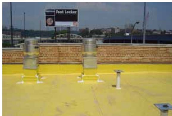
Yankee Stadium Building J Plaza restoration and greenroof assembly
