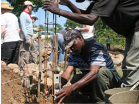
Building a foundation at the MPP eco-village.
