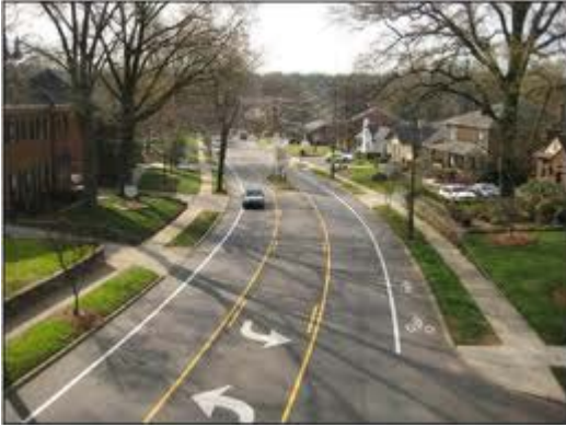
A road diet on this street in Charlotte changed a four-lane road to two lanes, narrowed the left-over travel lanes from 12 feet to 10 feet, and added wider sidewalks and bike lanes – all within the existing right of way.
