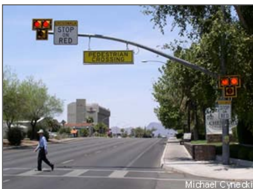
High intensity Activated crosswalk – HAWK – signals have been proven to dramatically reduce pedestrian crashes at mid-block crossings and intersections. They are included in the 2011 Manual on Uniform Traffic Control Devices (MUTCD).
