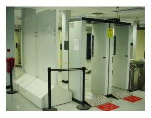
The shield wall that NPO built for Dresden was finished in a snowflake white to match the color of the other furniture in the area. The wall is mobile and made of solid lead with all casters connected.
