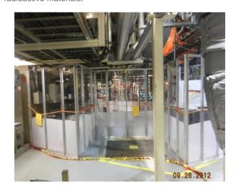
"The structure keeps stuff in place. Workers can't violate the boundary and accidentally pick up a contaminated lead blanket. Some material coming out of containment can be contaminated. Now it's contained inside walls," states Thompson. The system itself is kept clean – noncontaminated.
